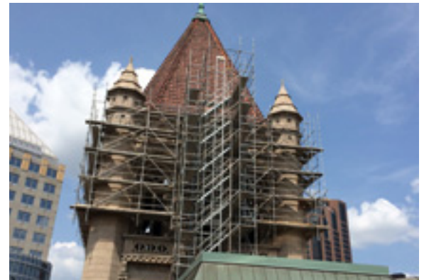
Scaffolding on Landmark Center's North Tower
